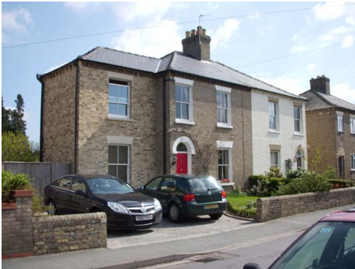
Extension to a semi-detached dwelling in the Histon Conservation Area that respects the form, scale and massing of the original. Note also the appropriate material selection and the well detailed sash windows.
