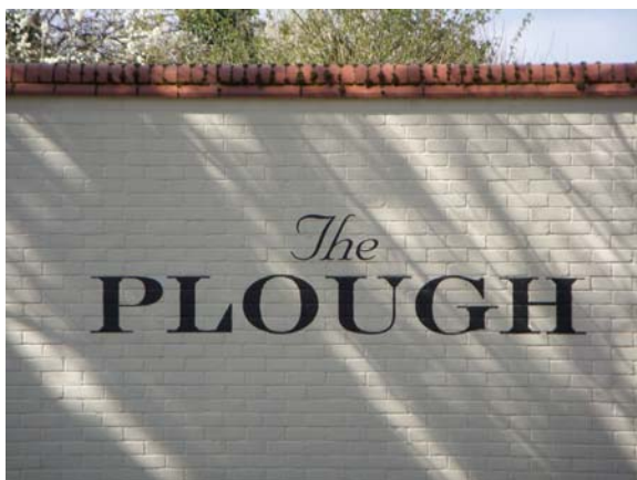
New painted sign on masonry wall in the Fen Ditton Conservation Area. Note also that it was not thought necessary to have to provide lighting to this sign
